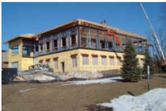
Progress on the Andres Center as of February 18, 2005
